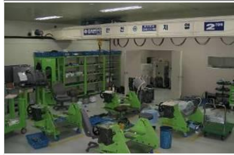
Dry Pump Center
